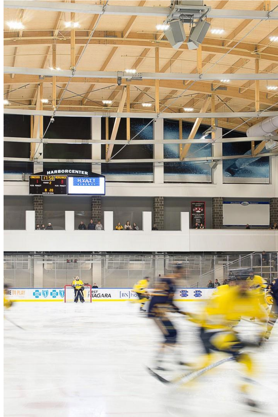
HarborCenter CLT + Glu-lam Roof Structure - Buffalo, NY
