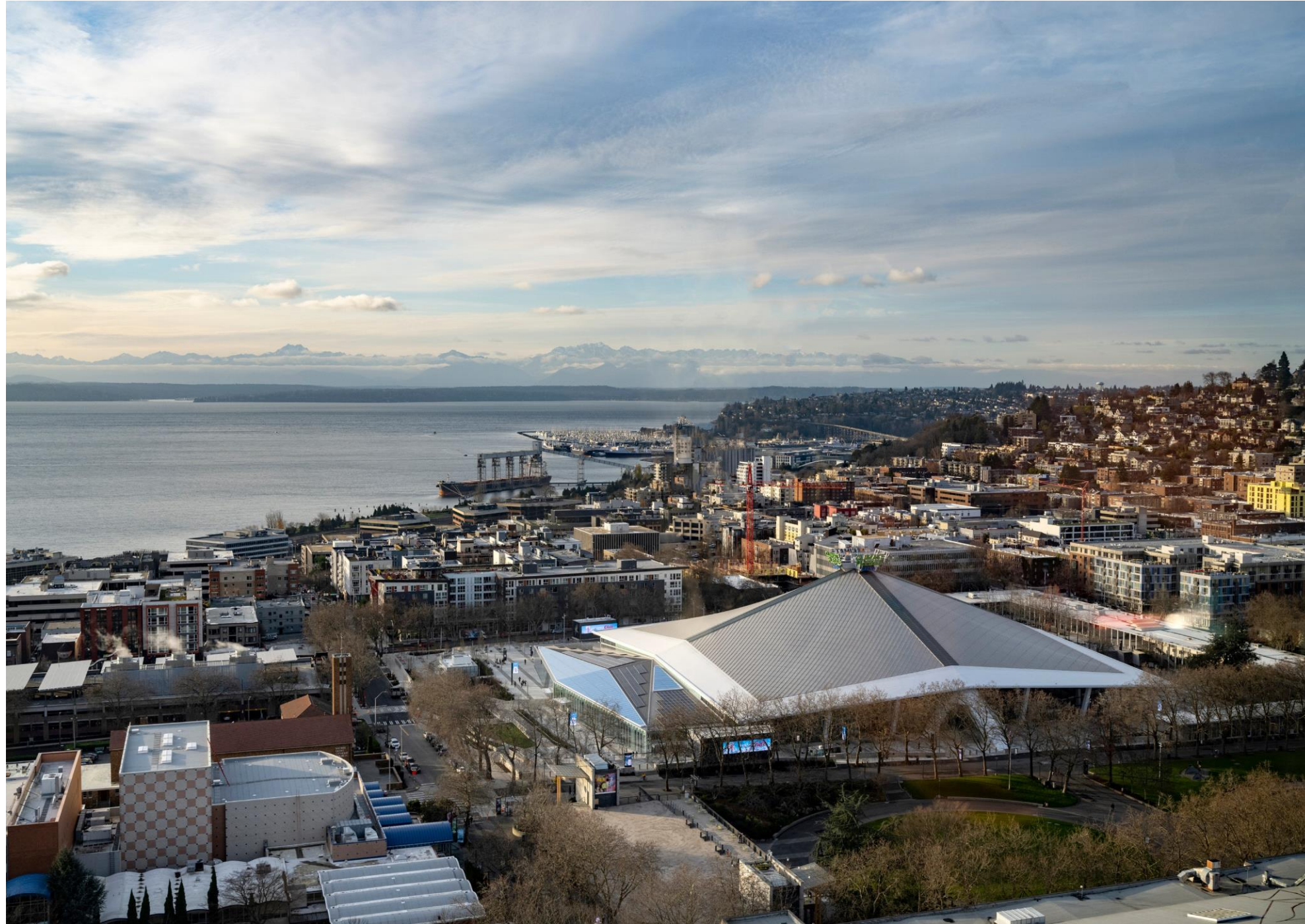
Climate Pledge Arena, surrounding neighborhood, and adjacent public park and cultural spaces - Seattle WA
